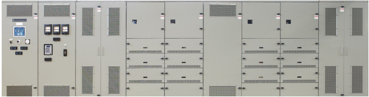
Totally redundant DECS-2100 system
